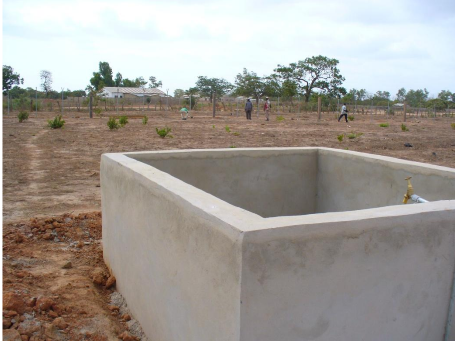
Figure 12 - Concrete Block Reservoirs, before matting was placed
