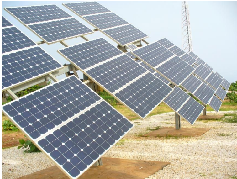
Figure 8 - Bwiam Hospital Solar Panel array with mounted tracking systems
