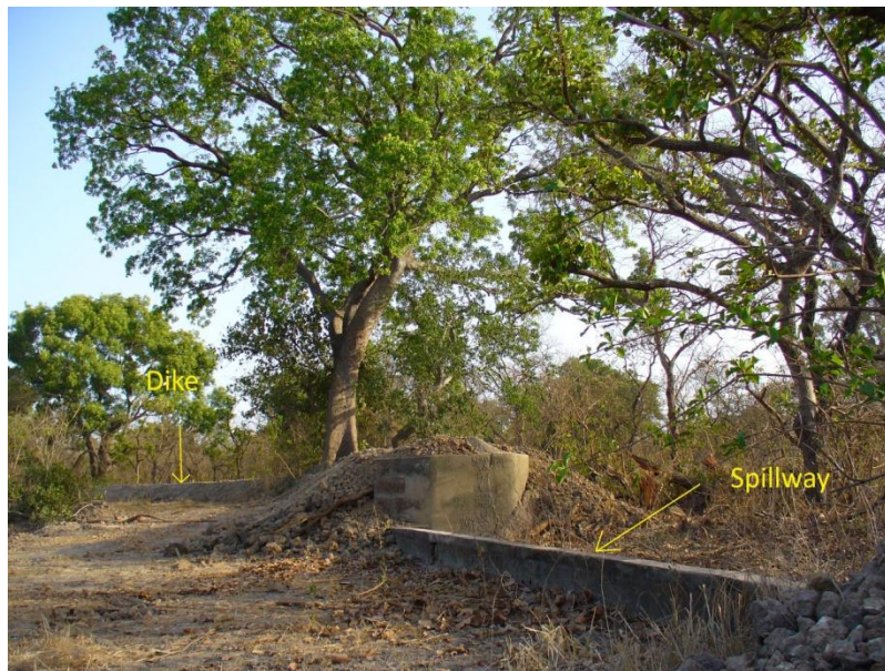
Figure 1 - Dike and Spillway recently constructed at Sohm
