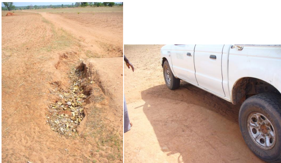
Figure 6 - Erosion beside the intersection Figure 7 - Example of the bund being eroded
