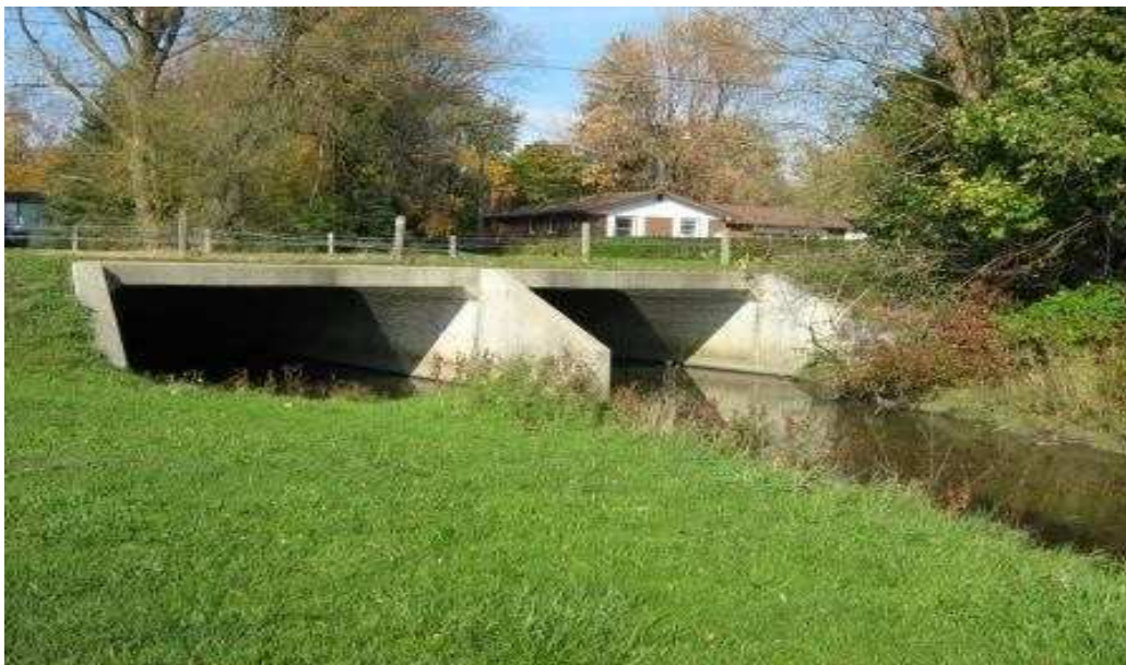
Figure 2.24 Parkhurst Ave Bridge (after City of London)
