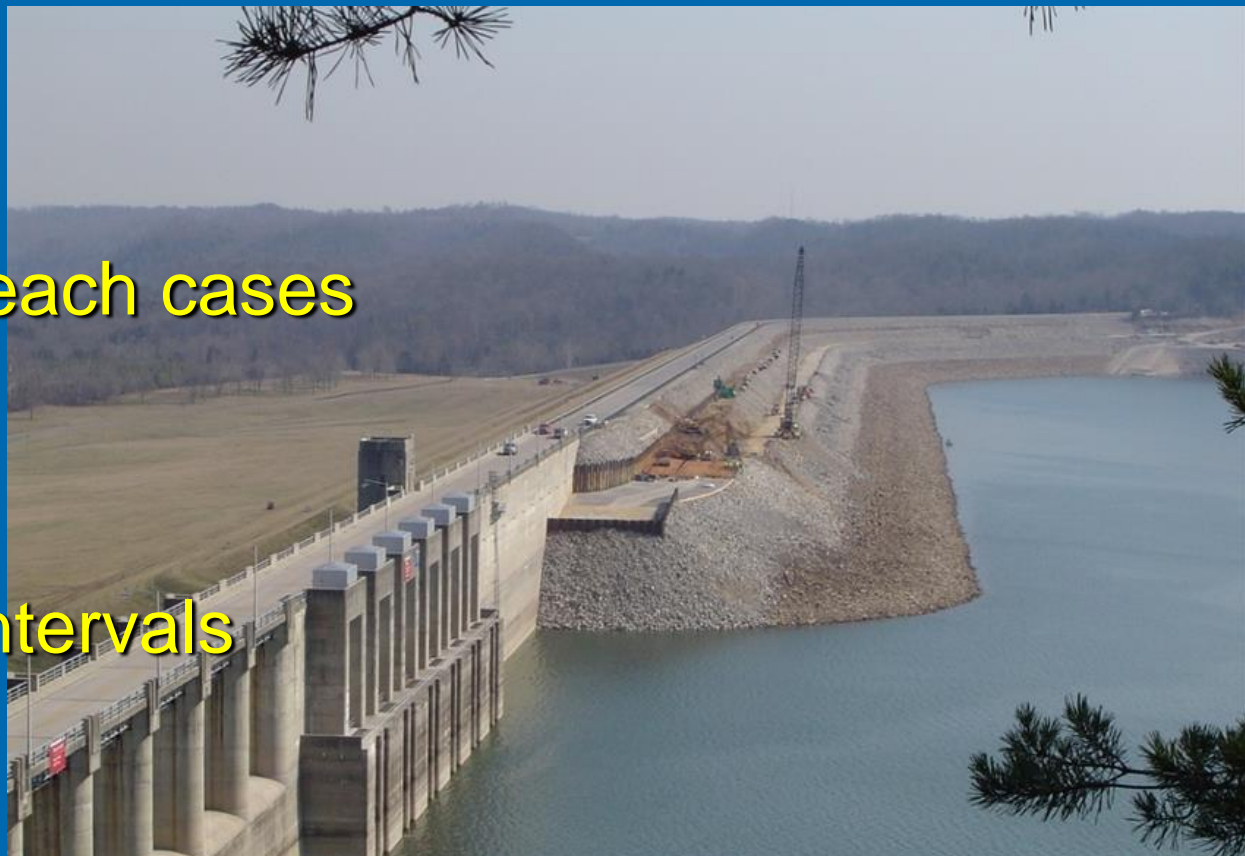
Wolf Creek Dam, KY
