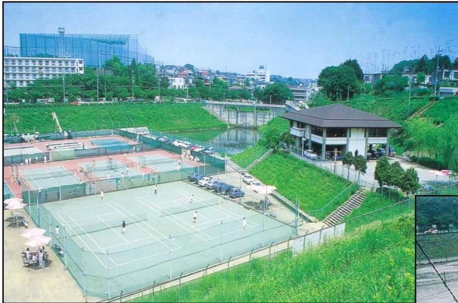
Kirigaoka regulating pond in the Tsurumi river basin (Kanagawa Prefecture)
