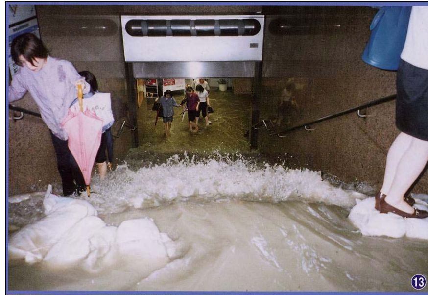
Flood water flowing into basement space by overtopping the sandbags
