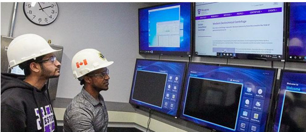
The drum centrifuge control room
