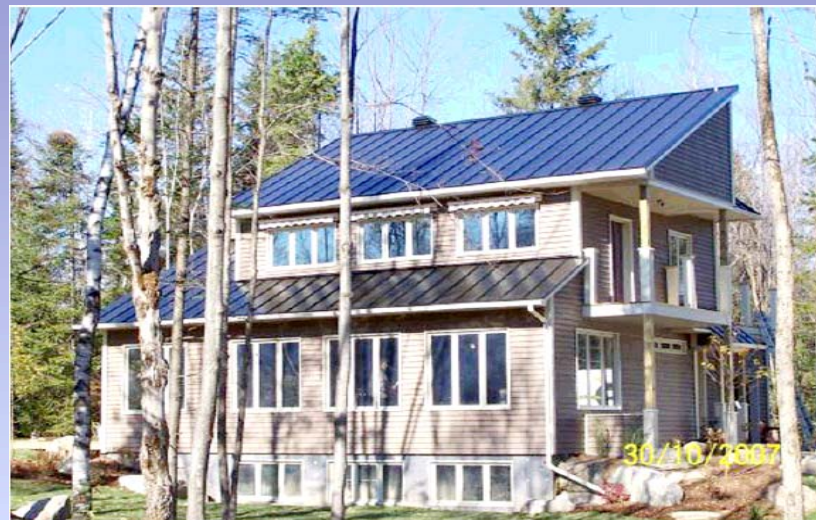
Photovoltaic-Thermal (PV/T) roof system
