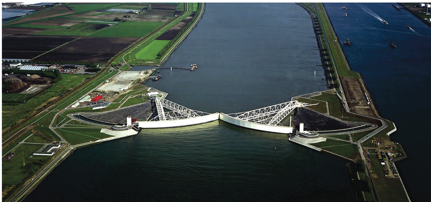
Fig. 3 — The Maeslantkering, a storm surge barrier in the Netherlands that automatically closes as needed, is one of the world's largest moving structures. Courtesy of holland.com.
