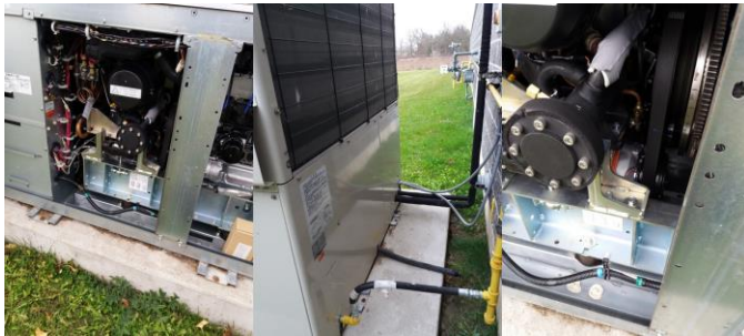
FIGURE 1. NATURAL GAS FUELED INTERNAL COMBUSTION ENGINE DRIVEN HEAT PUMP
