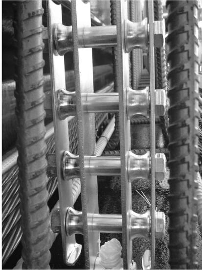
Figure 1(a): Hold-down device
