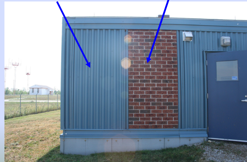
Exterior view of the control building
