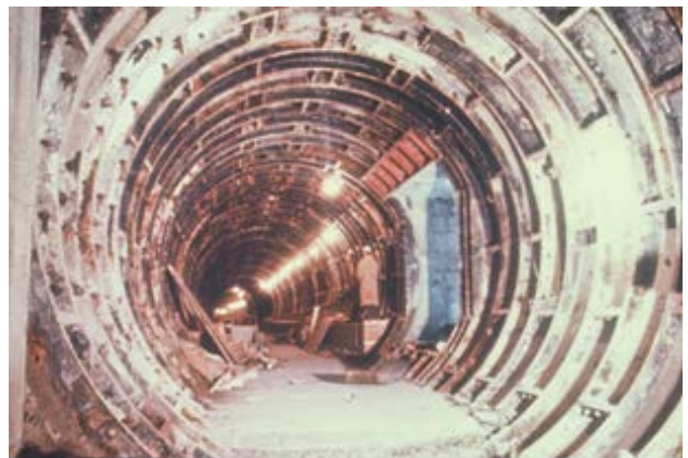
Figure 2. TTC Subway tunnel
