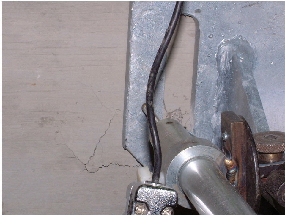
Figure 10 Cracks Observed at Displacement of 7.5mm (Test V1)
